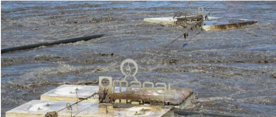
Mapal's floating fine bubble aeration system in full flow
