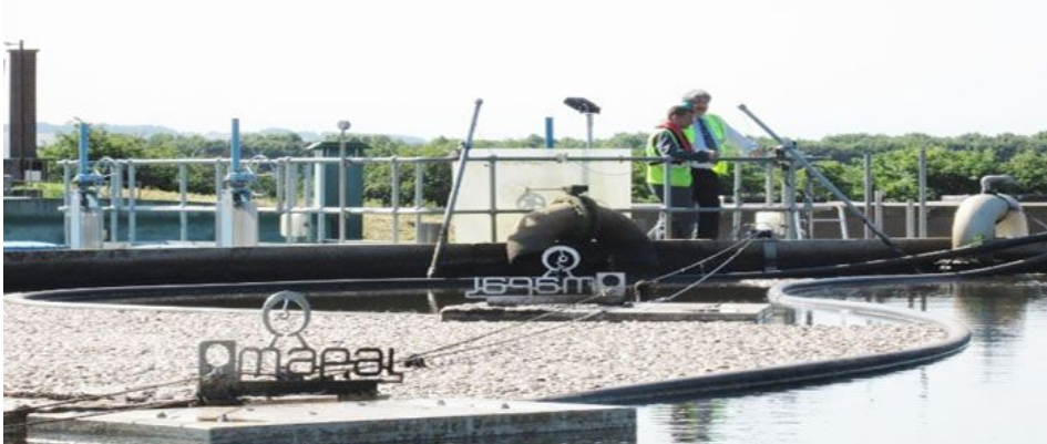
The floating modular system can reduce operational down-time by being easier to install and maintain
